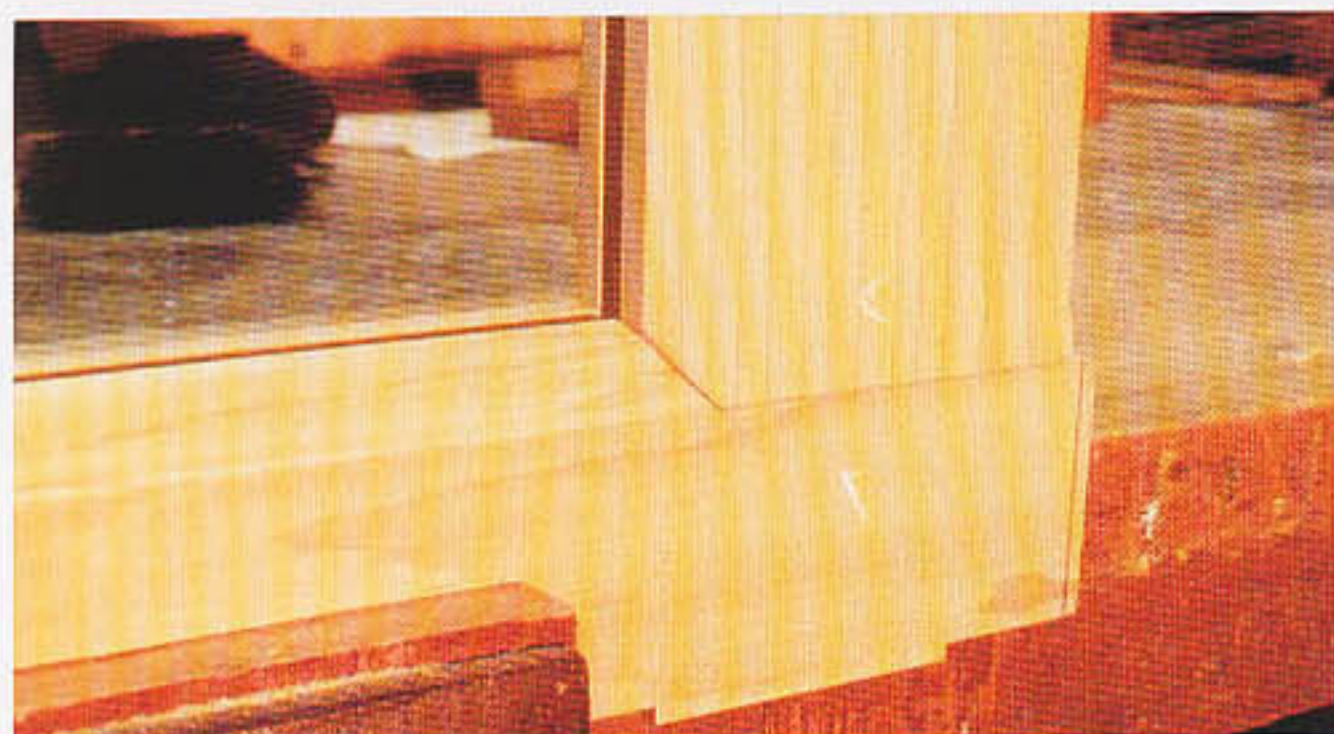
I ran off the mouldings and cut the panel groove with the spindle moulder, and then cut the joints
